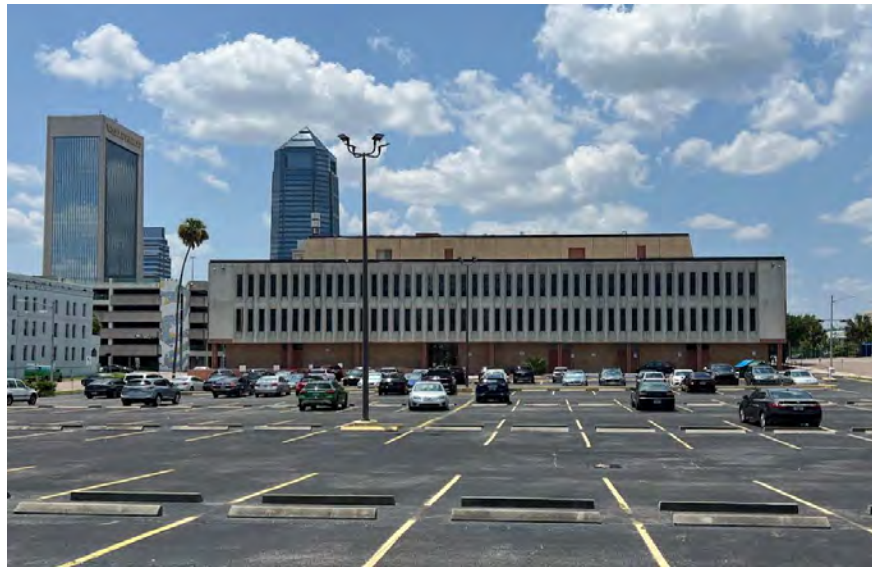
West view of the Fuller Warren Building
